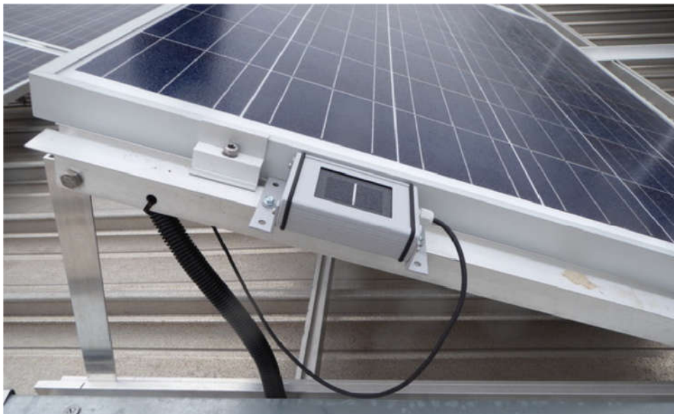
Installation of M&T Si Sensor in a Solar Plant
